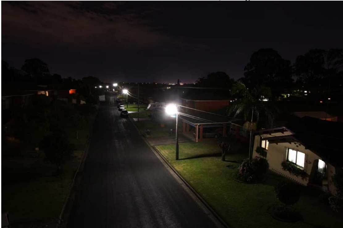
Before – Twin 20 fluorescent luminaire - Oak Drive, Georges Hall
